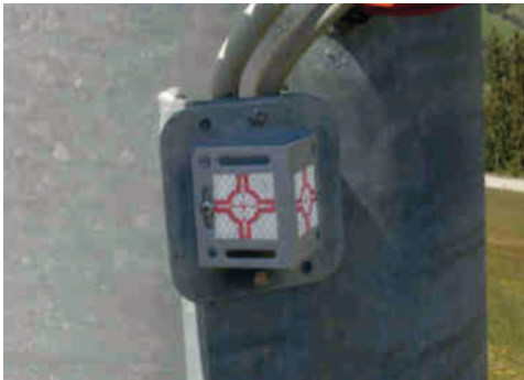
Measuring point on the ski lift support
