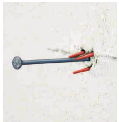
Elastic "stubs" for securing the surveyed measurements are securely marked until plastering work is completed.
