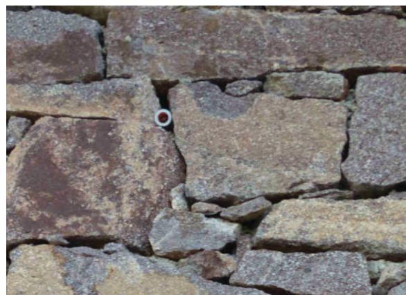
RSM P12 – Monitoring on the brickwork
