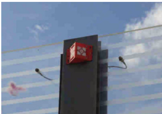
Observation of sound barriers walls
