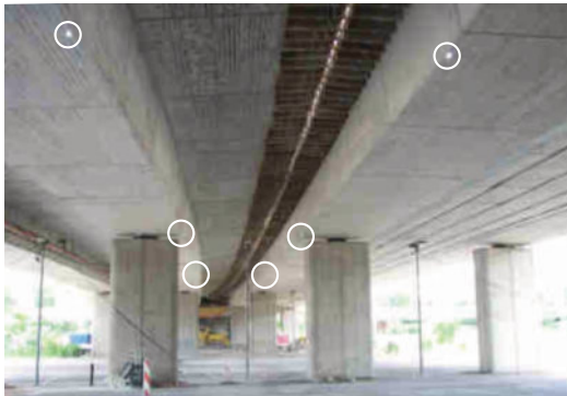
Observation of bridges
