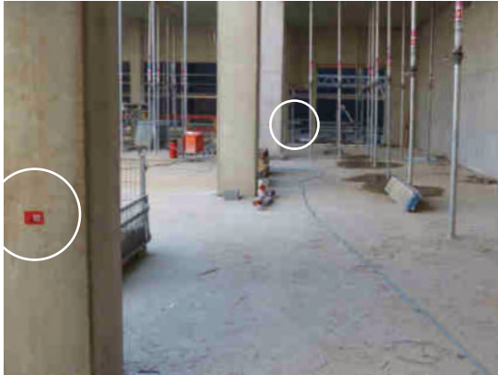
RS30r in industrial construction: Documentation of heights and axes in one product.
