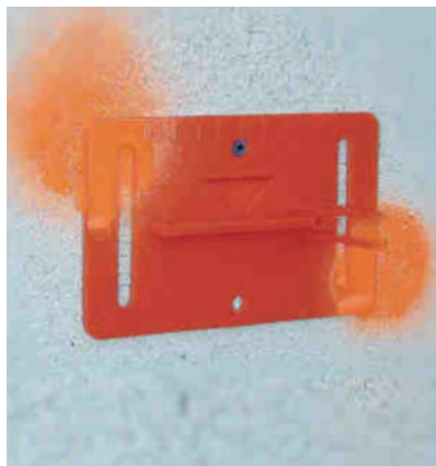
RS21r glued, fastened, and sprayed over with colour to prevent tampering.
