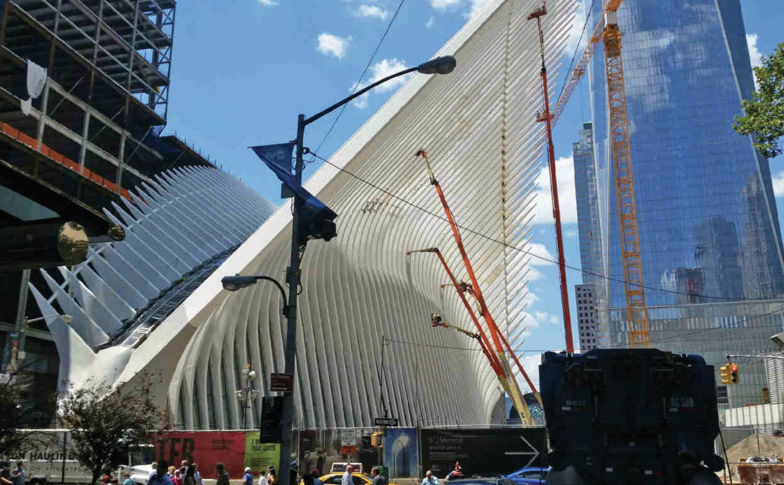
Underground Station, World Trade Centre in New York City
