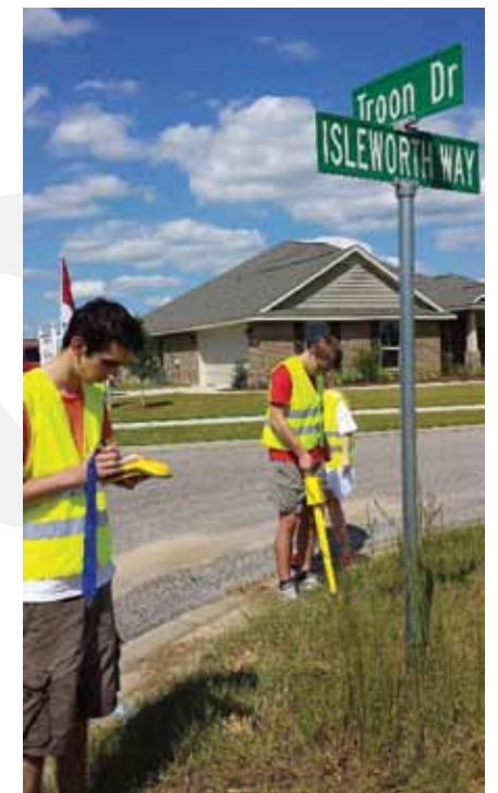
GPS, maps and landmarks are used to get close to the buried InfraMarker magnetic RFID tag which is found with a magnetic locator. Photo courtesy of Auburn University Geospatial Research and Application Center.
