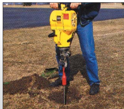
The rod monument is driven into the ground, a section at a time, to refusal*. The top of the last rod should be about 6 inches (150 mm) below the surface. *See page 15
