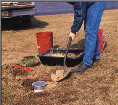
The hole and pipe are carefully back-filled with sand. The top 12 inches (300 mm) of the hole (OUTSIDE of the PVC Pipe) are back-filled with concrete.
