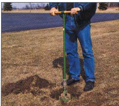
A 12 inch (300 mm) hole is augered to a depth of about 3 1/2 feet (1050 mm).
