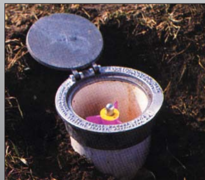
A 6 inch (150 mm) diameter PVC pipe 3 feet (915 mm) long, with access cover glued on, is placed over the finned sleeve (pipe should not touch the fins). Back-fill (INSIDE the PVC Pipe) with sand.
