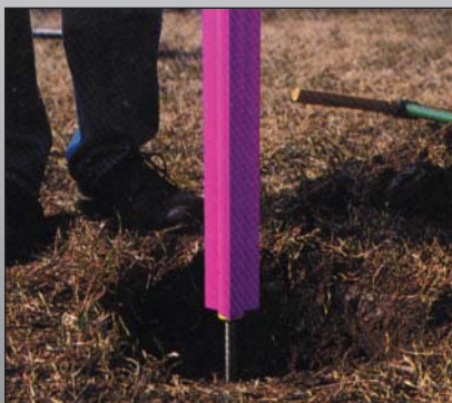
The finned sleeve (filled with grease) is placed over the rod and the datum point added (or filed onto the rod end).
